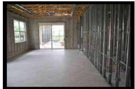
Complete Remodel - Venice, FL
