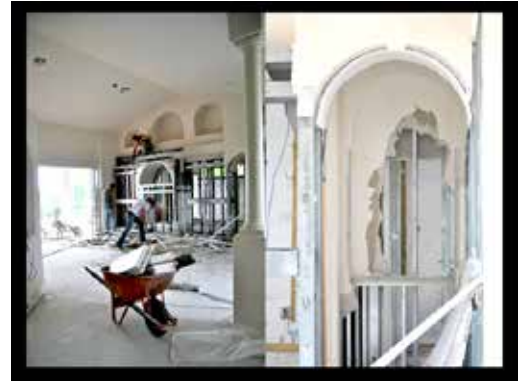
Complete Remodel - Venice, FL
