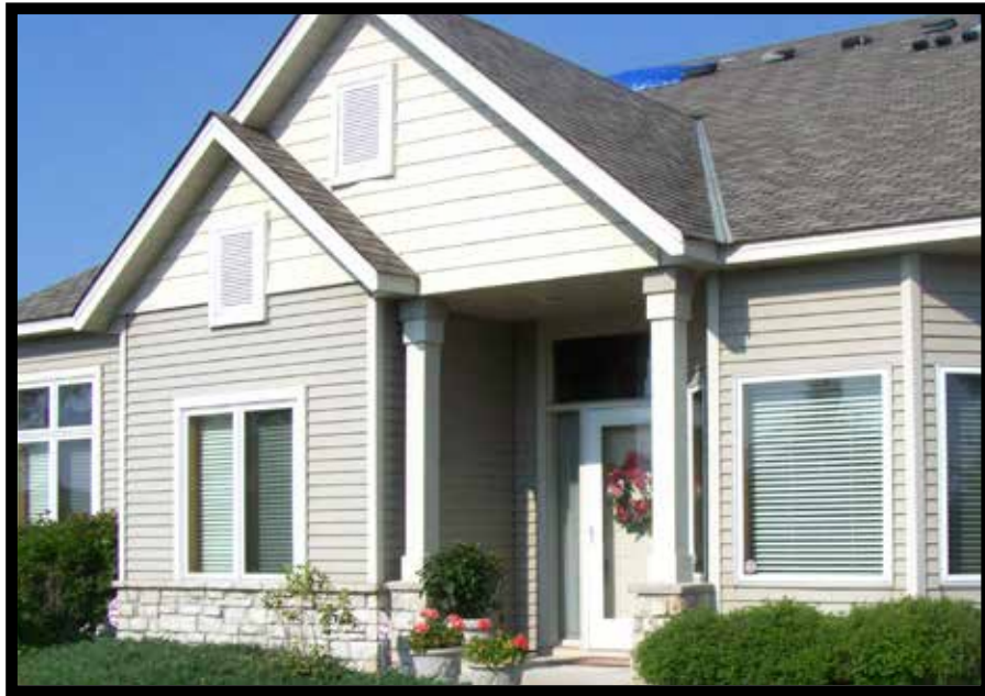
Exterior Remodel - Harrison Place, Plymouth, MN
